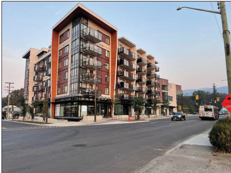
Residential and Town & Village Centre Development
