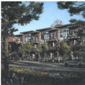
SITE 2: VIEW ALONG MT. SEYMOUR PARKWAY
