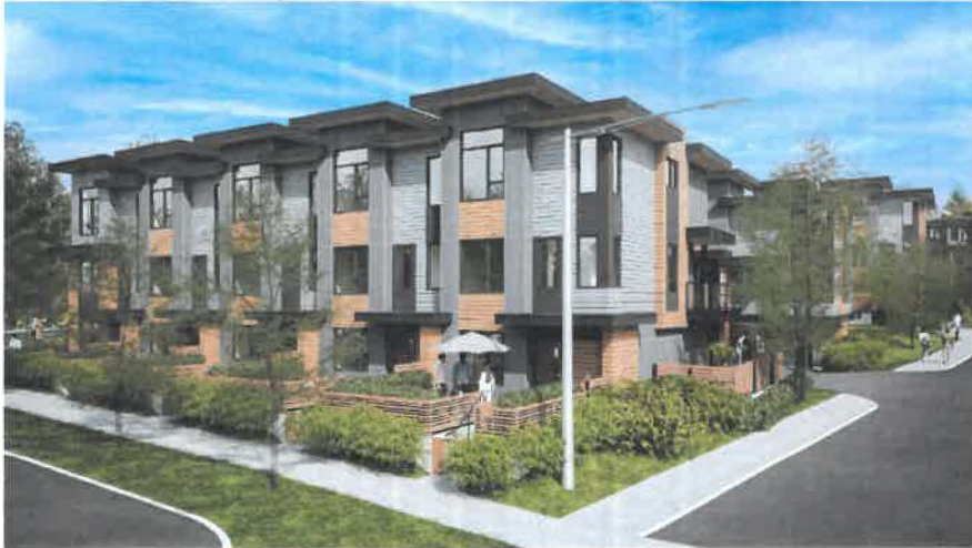
BUILDING 1 - VIEW FROM LYTTON STREET & LOWER RING ROAD
