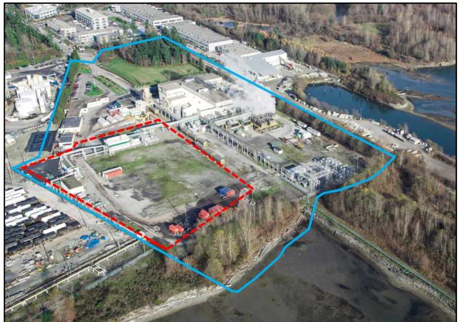
Looking north-east across the subject property outlined in blue, the red dashed line shows the approximate location of the proposed hydrogen facility.
