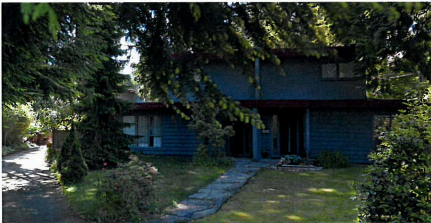
Figure 6: Duplex with side by side units at 3703 & 3711 Bluebonnet Rd., North Vancouver
