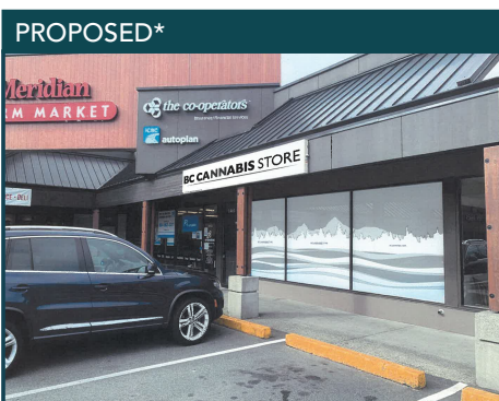
*Provided by applicant for illustrative purposes only. The actual development, if approved, may differ.
