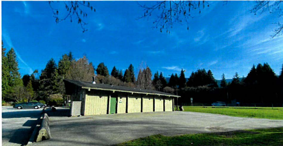
Figure 2: Eldon Park Field House is nearing the end of its functional life and provides an ideal site for a shared-use field house and child care facility.
