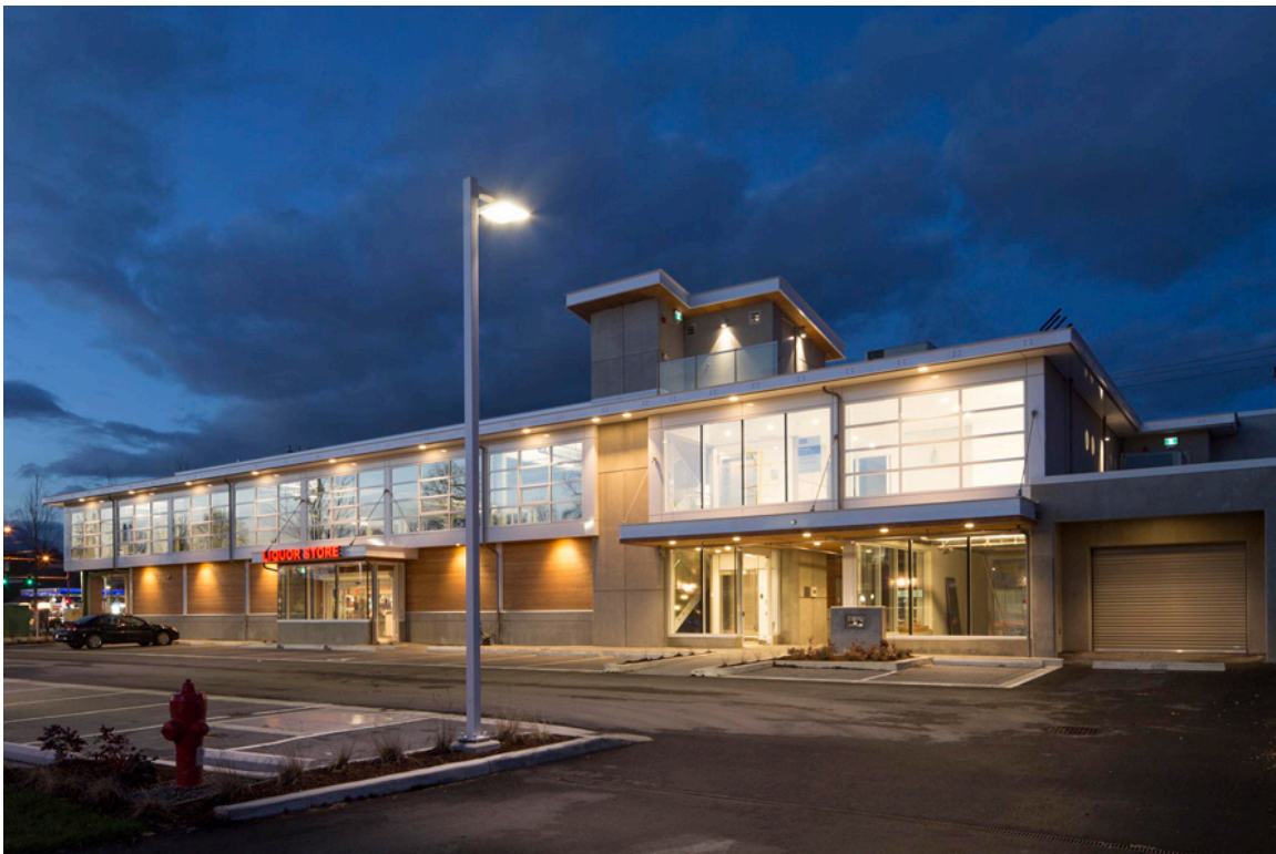
1520 Barrow Street. The CRS is proposed to occupy the ground floor unit on the right hand side.
