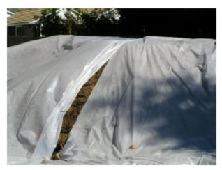
Soil stockpiles and exposed soil must be covered with plastic or other suitable erosion control products (vegetation, biodegradable fabric, etc). This protects exposed soil on slopes or boulevards from wind and water erosion. The Soil is also protected from becoming saturated with water making it difficult and more expensive to handle. Vegetation covers such as grass, wildflower seed mix or shrubs can also be applied to provide longer term protection.
