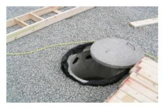
A sediment trap or sump is a co llection area where sediment laden water is temporarily stored, allowing sediment to settle out before the water is discharged. Line the outside of the sump with clean gravel and then wrap the concrete sump with a heavy geotextile fabric.
