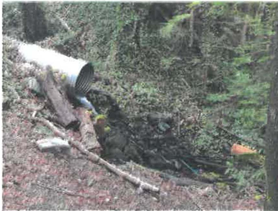
A stormwater outfall releases into a naturalized side channel of Mackay Creek.
