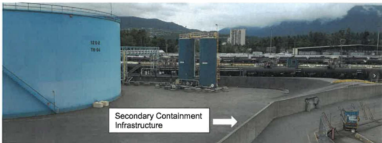
Example of existing spill containment area and enclosure
