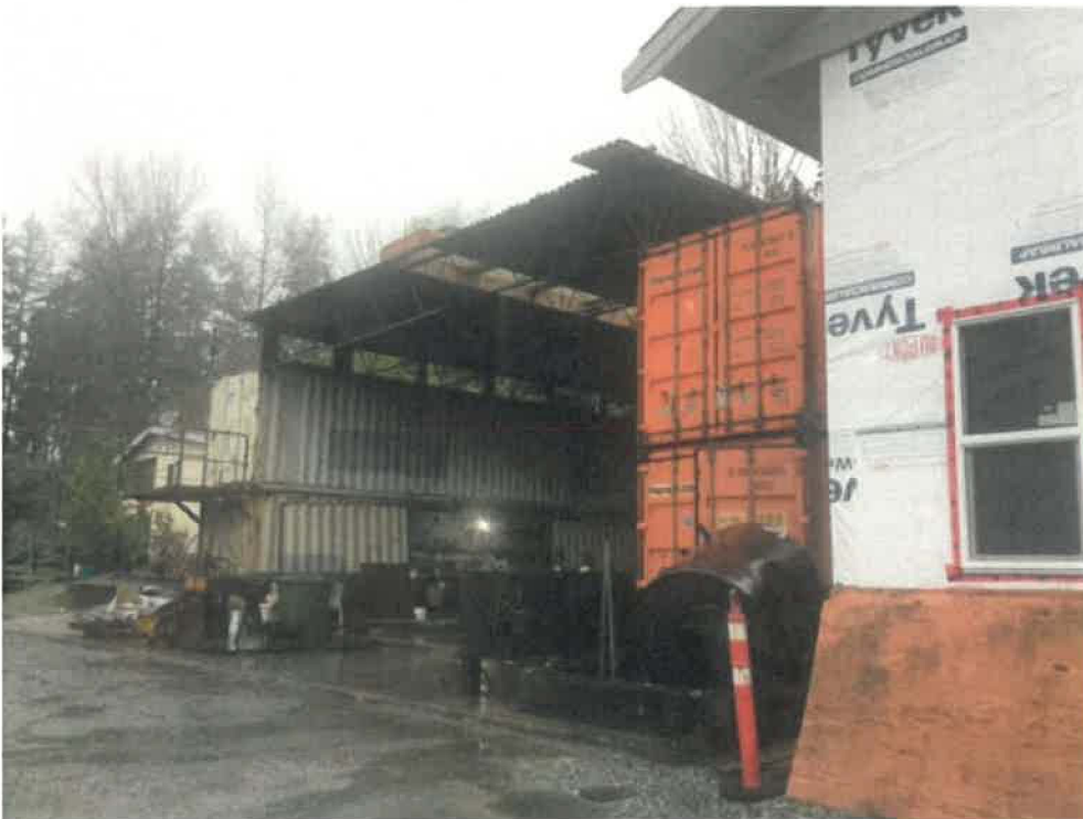
Steel-trussed roof structure over shipping containers
