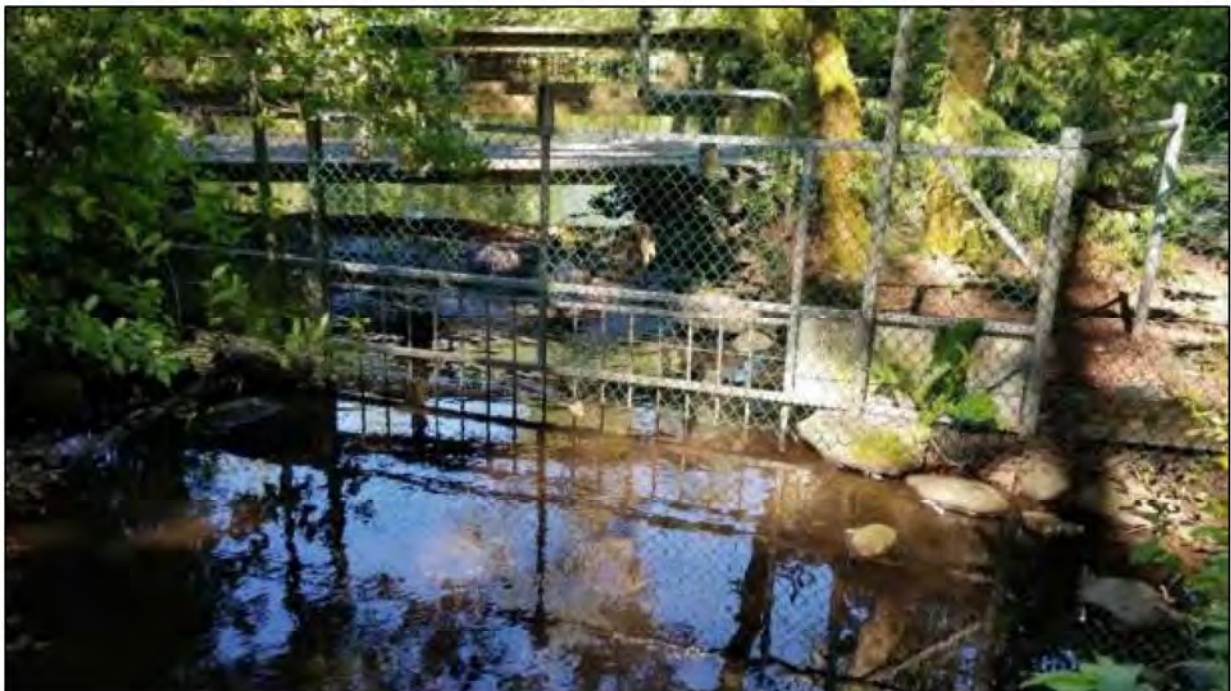
Photograph 10: Looking northeast towards the rock and concrete sill at the Maplewood Pond outlet, which presents a partial barrier to fish passage.
