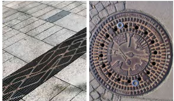
Examples custom designs for manhole cover and drainage channel cover
