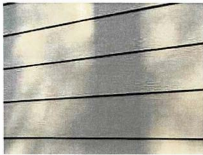
1 FIBER BOARD BEVENT HORIZONTAL LAP JOINTS
