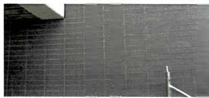
5 BRICK VENEER (STACK BOND)
