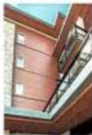
4, 14 LONGBOARD (1/2 V GROOVE) HORIZONTAL SIDING AND SOFFIT
