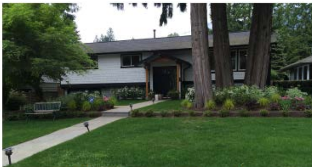
Older house on a large lot
