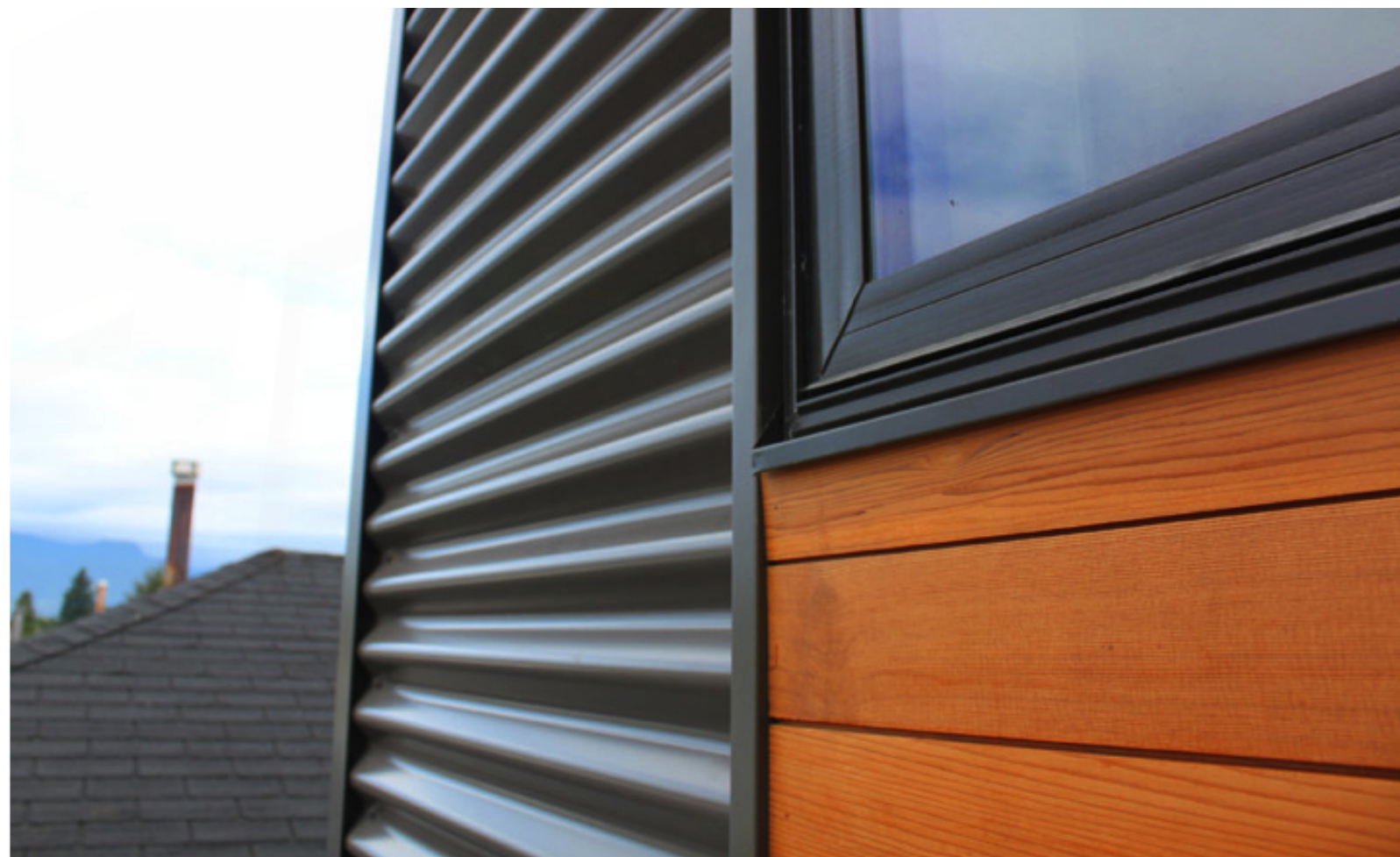
HardiePlank Lap-Siding @ Siding Change and @ Window Sill
