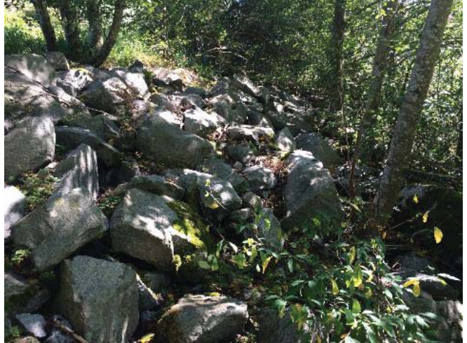
Photo 10 Riprap bank protection along Lynn Creek left bank, facing west
