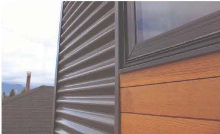
HardiePlank Lap-Siding @ Siding Change and @ Window Sill
