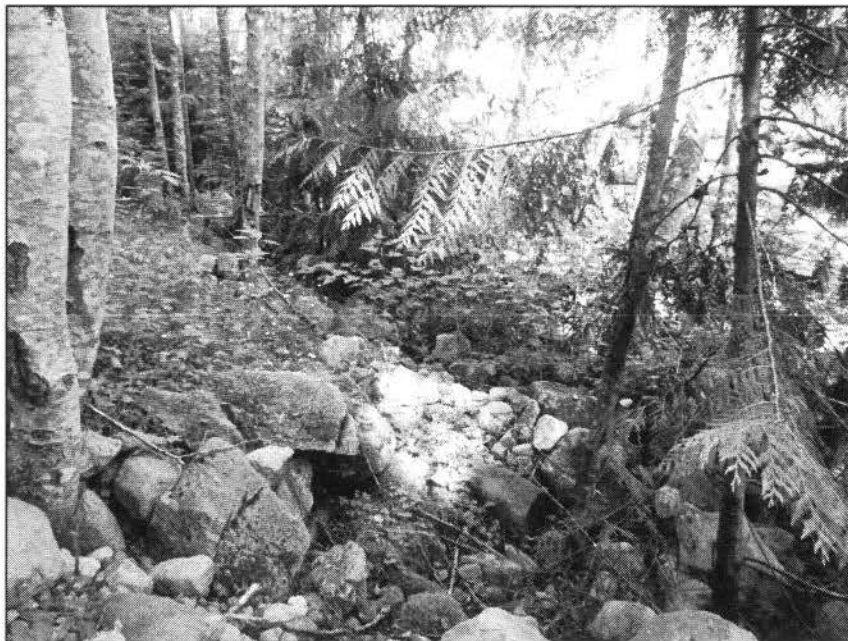
Photograph 6 View from the walking trail at the approximately 0.50 to 0.75 m diameter riprap along the right bank of Mosquito Creek at the toe of the slope (July 8, 2013).
