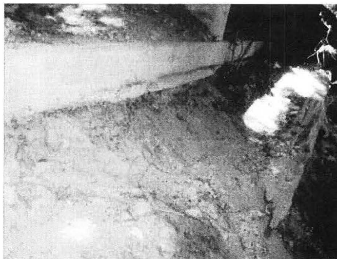
Photograph 2: erosion at south side of house foundation and old log supporting ravelled soil.
