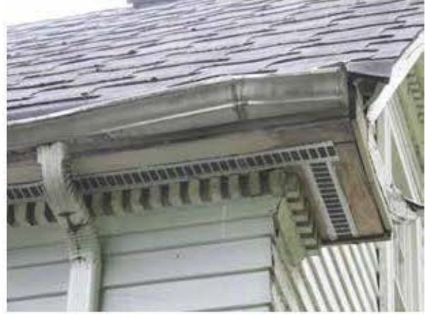
Detail photos showing typical deteriorated condition of asphalt-shingled roof along gutter and eaves.
