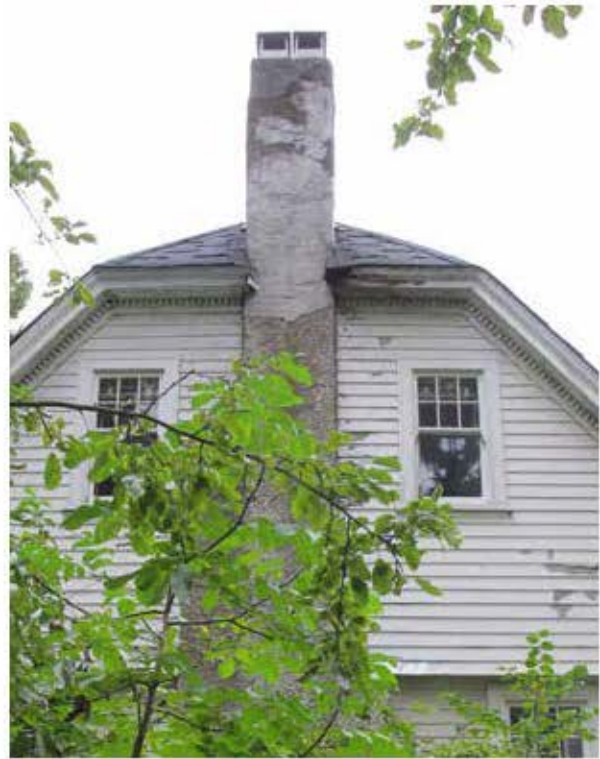
Typical existing condition of exterior brick chimney with later rough-cast stucco.
