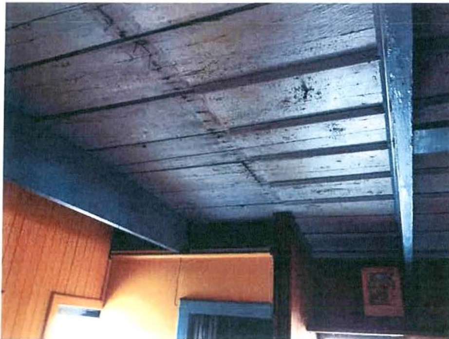
Photo 6 – Wall and roof joist has been removed
