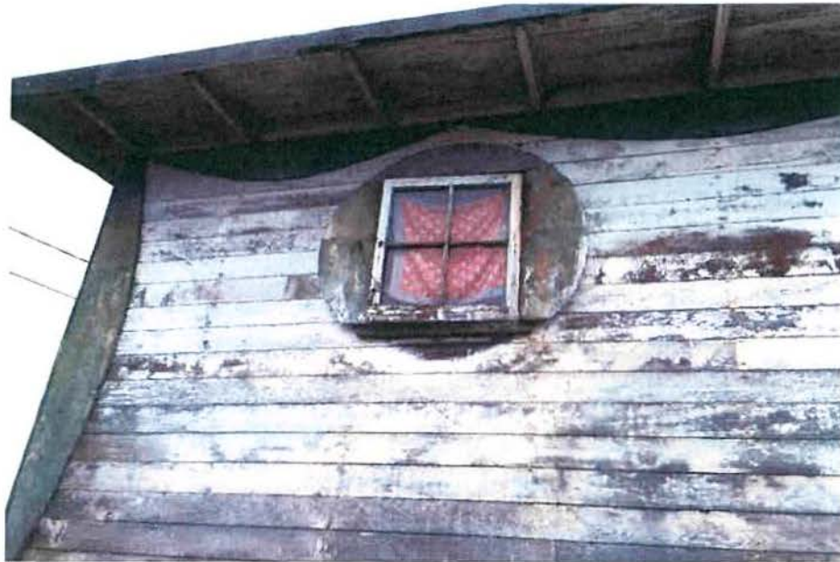
Photo 3 – Weathered siding and wood detailing trim
