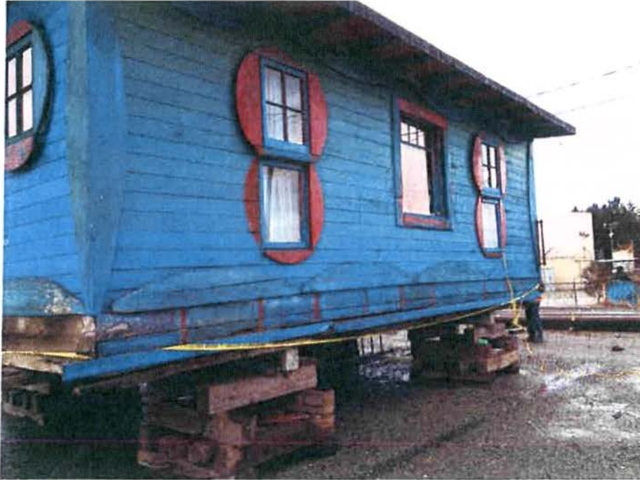
Photo 1 – 'Blue Cabin' - side elevation showing timber cribbing supports
