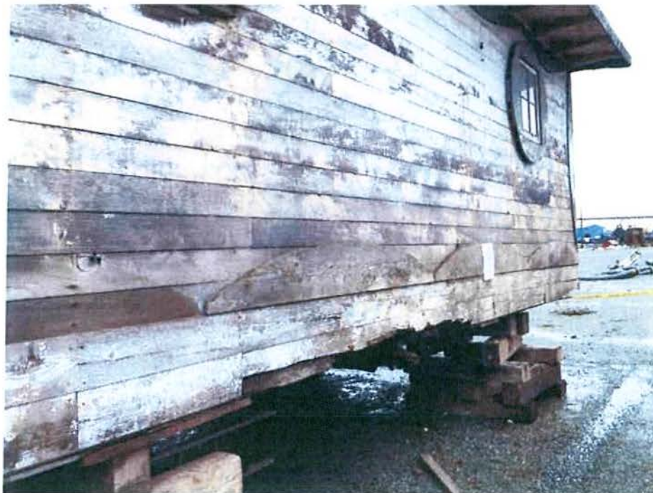
Photo 4 – Rotted siding and box joist
