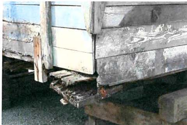
Areas of structural deterioration in the support beams under the cabin. (Andrew Todd)
