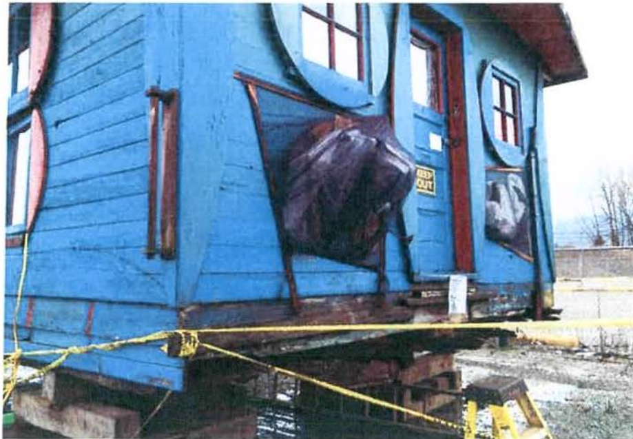
Photo 2 – End elevation - box joist rotted; old dock lumber remains below cabin
