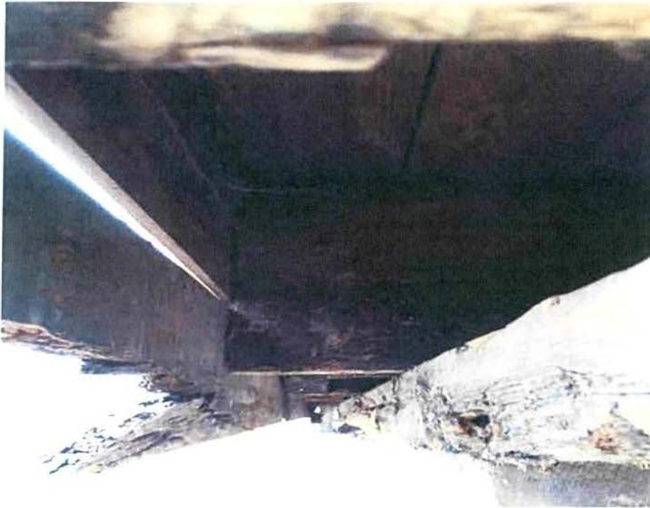
Photo 5 – Box joist and ends of floor joists rotted; floor boards generally sound
