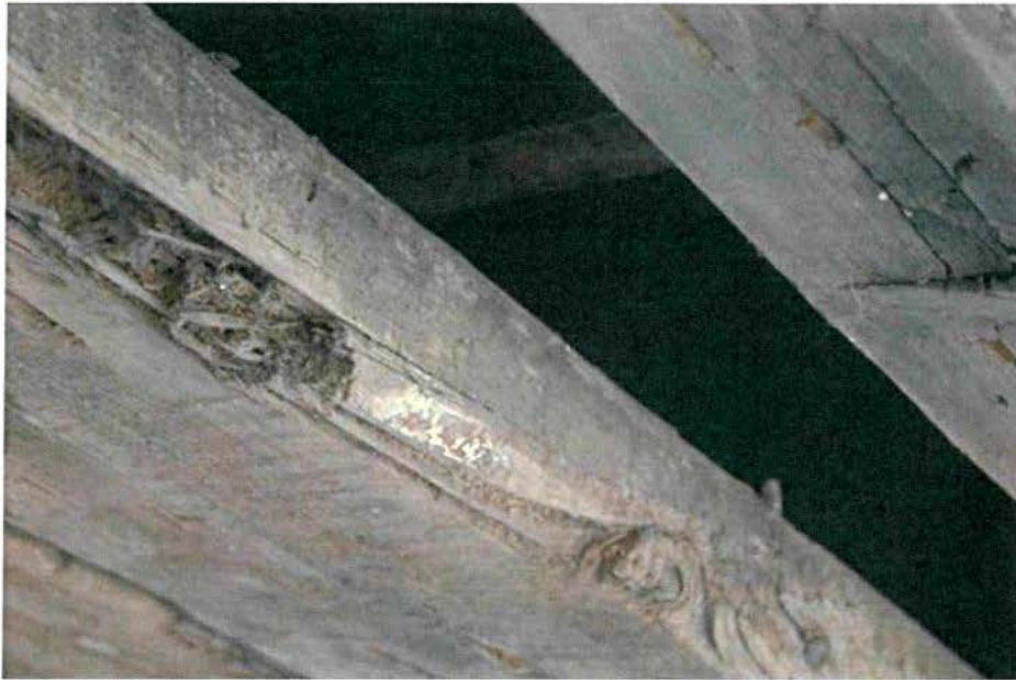
Detail of brown cuboidal fungal deterioration, frass, and small flight holes of insects, possibly furniture beetle or carpenter ant. (Andrew Todd)
