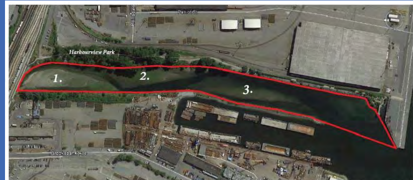
Figure 8: Aerial image outlining the estuary (red polygon) with the main 4 gravel bars labeled 1-3. The proposed aquatic habitat improvements will focus on gravel bar #2 and the riparian habitat improvements alongside and throughout Harbourview Park. (Image adapted from: Google Earth. Image date: 14-July-2014.)
