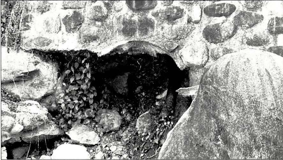
Photograph 7. Erosion beneath concrete wall at outlet of drainage pipe.
