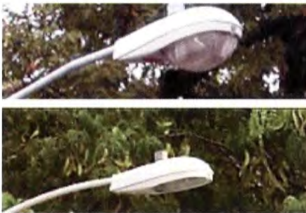
Old drop lens and new flat lens (photo: BC Hydro)
