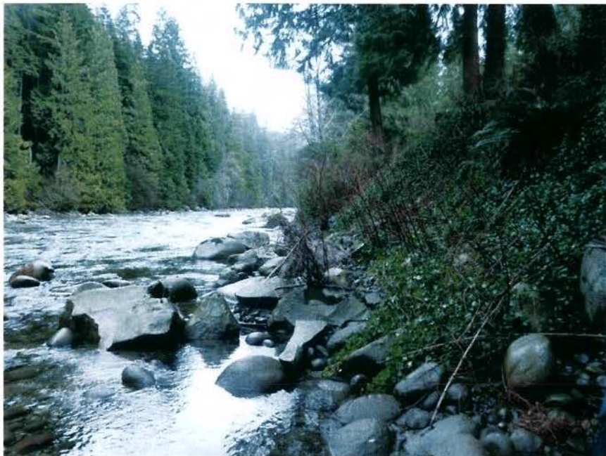
Photo 1. Large boulders (angular) placed at the bottom of the toe of bank, providing stability and limiting the risk of erosion. View looking from upstream from southern edge of property.
