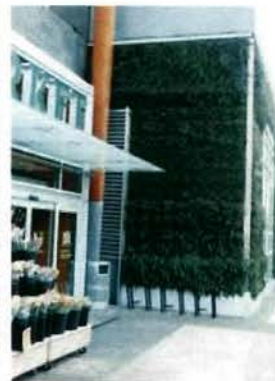
FIGURE 44 Integration of a green wall and passive shading devices
