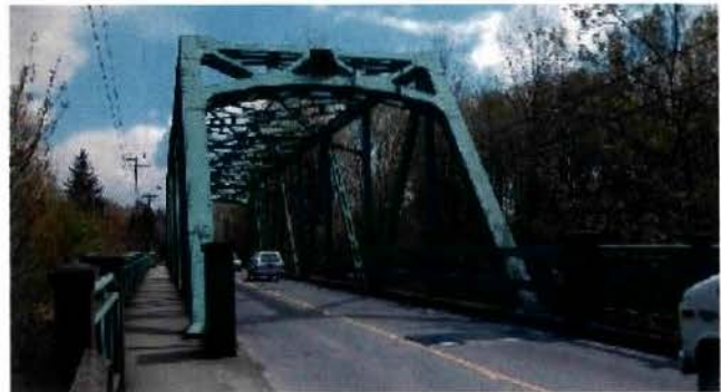
Keith Road Bridge, facing west
