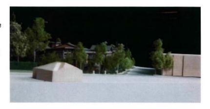
Due to the slope of the land, the north end of the building (adjacent to the single family lots on Ridgewood Drive) will be approximately two storeys above the existing grade (see section drawing below). A shadow analysis indicates that the building will not cast adjacent buildings into shadow.
