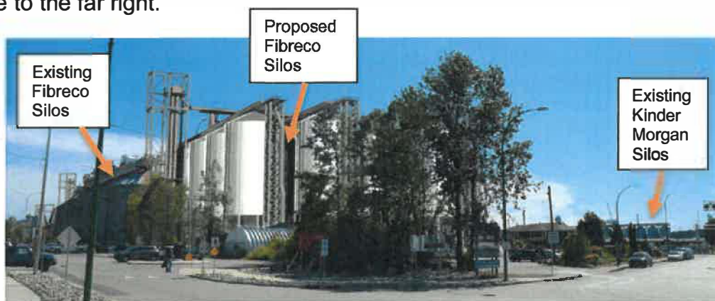
View from McKeen Avenue and Pemberton Avenue
