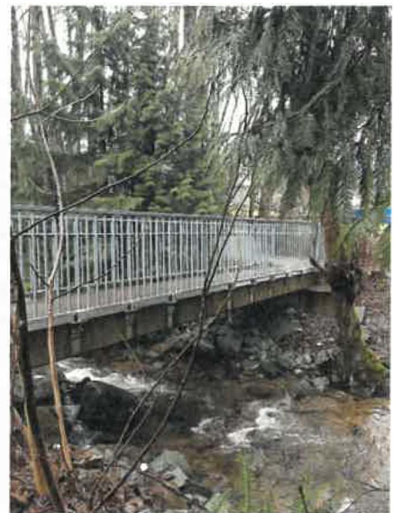
Bridge to Baird Road over Hastings Creek
