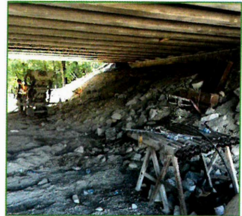
Beginning of drilling the new retaining wall under the Highway 1 Overpass
