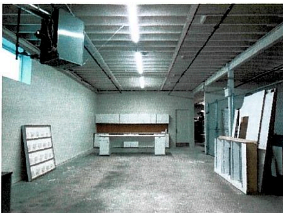
Collection storage warehouse renovation in progress.
