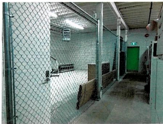
Collection storage warehouse renovation in progress.
