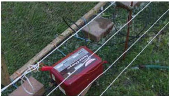
I ran water on the ground rods to make the soil more moist and help with putting a good charge on the fence.
