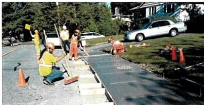
Concrete pouring for new sidewalks
