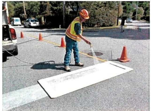
Crosswalk marking renewal
