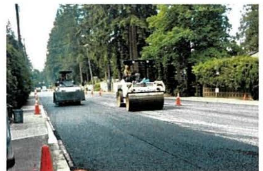
Paving of Capilano Road after water main work
