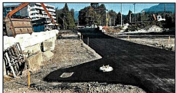
Barrow Street connection
