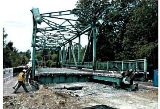
Old Keith Bridge being dismantled on roadway.
