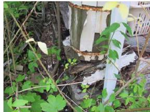
Example of dry rot on side porch column base
