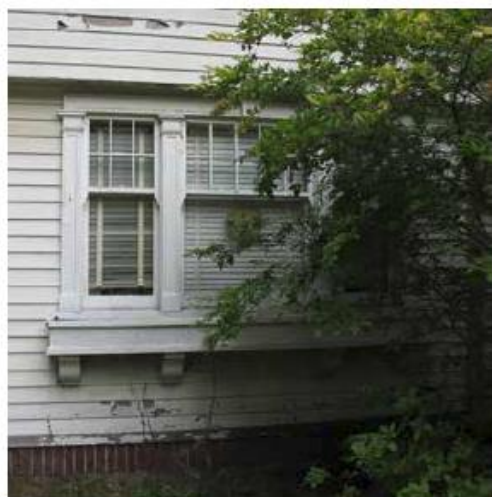
Tripartite 6-over-1 with 10-over-1 centre unit true-divided double-hung window
