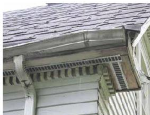
Detail photos showing typical deteriorated condition of asphalt-shingled roof along gutter and eaves.
