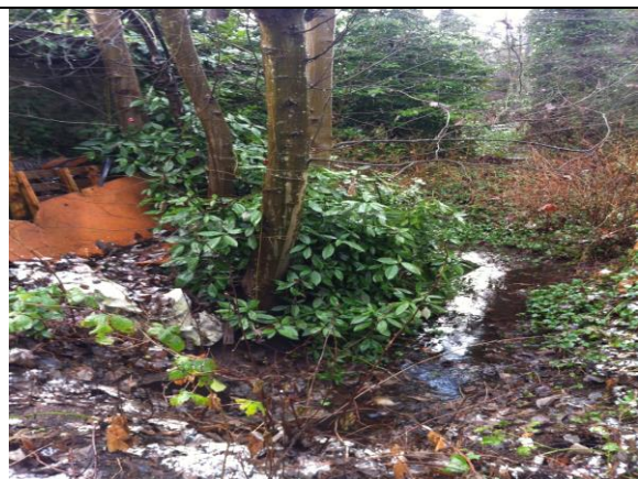
Photo #2: Ditch along western edge of property in LANE R.O.W. looking south along lane R.O.W.
