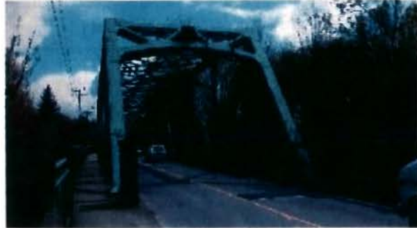
Keith Road Bridge, facing west
