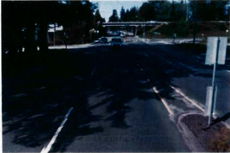
Lynn Valley Road, facing south
