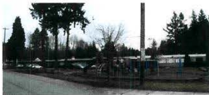
6. VIEW TOWARDS SCHOOL PLAY GROUND
