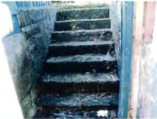
Missing handrails
