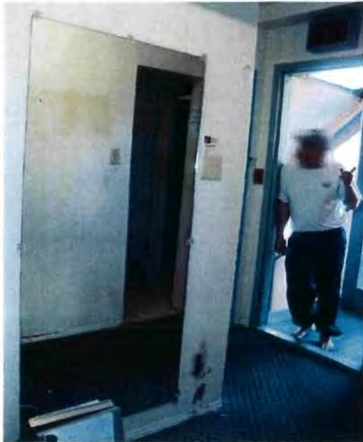
Mirror near exit, mounted on public corridor wall creates potential egress confusion
