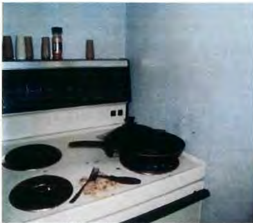
Cooking range beside combustible wall finish
