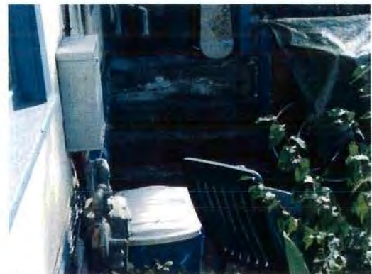
Missing handrails
