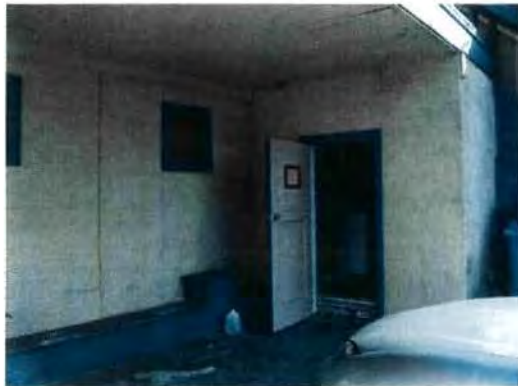
Wired glass in light aluminum frames exposing exit door
