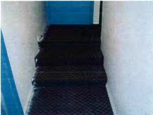
Missing handrails
