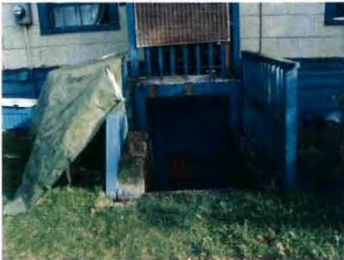
Missing handrails
