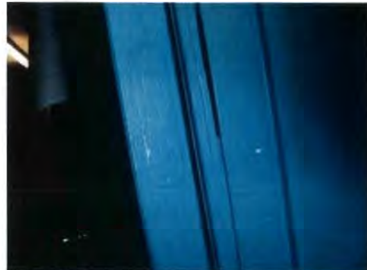
Fire test labels painted over
