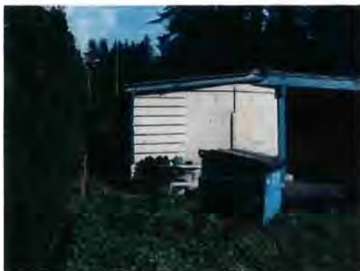
Proximity of the north face of the building to the north property line
