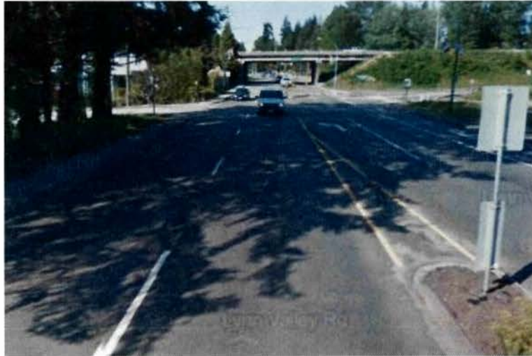
Lynn Valley Road, facing south
