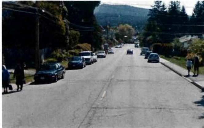
West 29 th Street, facing east
