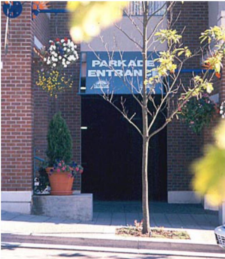
Parking entry incorporated in street facade
