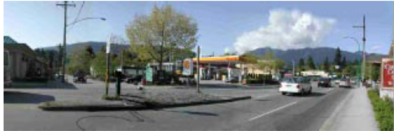
Capilano Road at Curling looking north as it exists today.
